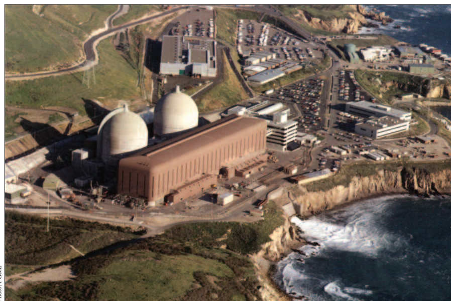
PG&E’s Diablo Canyon plant, located at Avila Beach, Calif.
